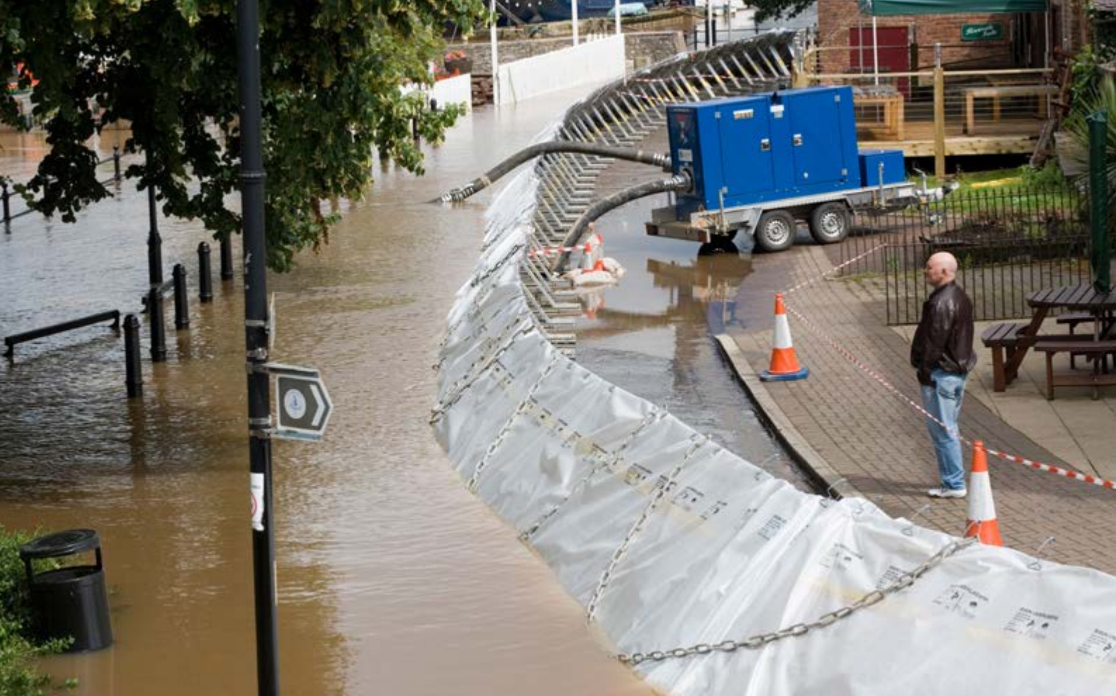
Flood barriers alongside the flooded River Severn in Worcestershire Mark Boulton / Alamy
